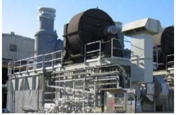
NATCO CHF controlled-heat flux heater with 1,000-degF process outlet temperature capability.
