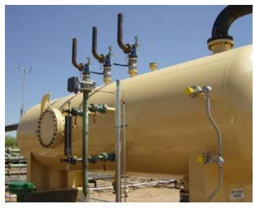
Valves used during separation must be designed to last since the process fluids may still be corrosive and contain abrasives and chemicals.
